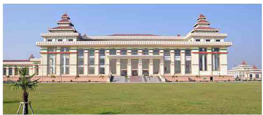
► One of the Myanmar government buildings in Naypyidaw.
